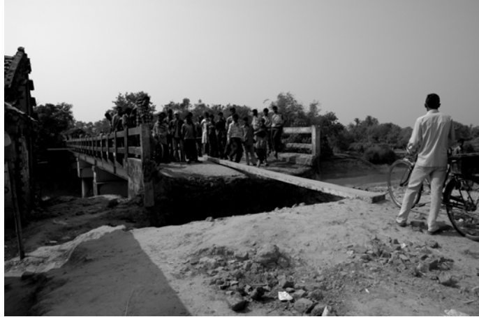
A trench by Talpatti bridge
